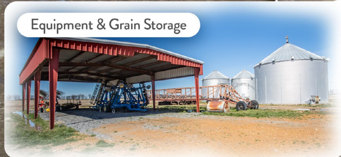
Equipment Storage Shed
